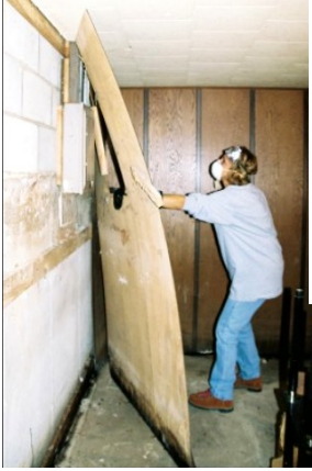
Tami Brunke rips out paneling from the basement walls.
