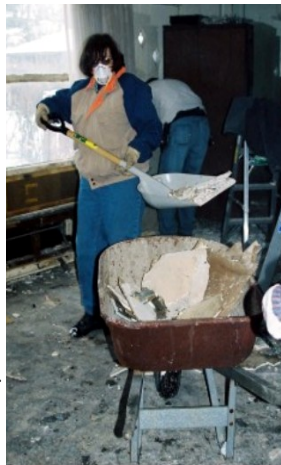
Paul Krilich guts the ceiling that was moldy from water seepage after the tornado in August caused roof damage.
