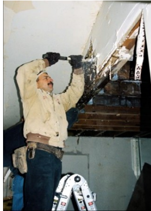
Paul Krilich guts the ceiling that was moldy from water seepage after the tornado in August caused roof damage.
