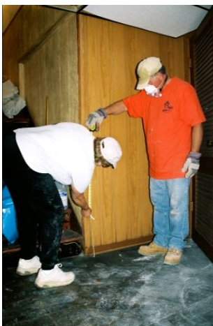
Jack Quinn assesses mold damage with homeowner, Amparo, East Chicago resident. Linda Burns and Joe Kovacs (below) measure cutline on paneling.
