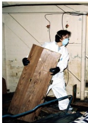
Karen Ditola hauls furnishings out of the basement.
