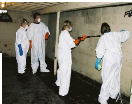
Sharon Majchrowicz and Alan Smith admire Laurie Rutkowki's power-washing technique as Gail Hartsough scrubs the bleach water on the walls.
