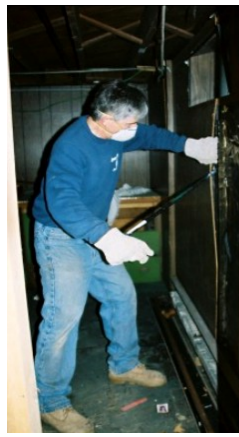
Joe Melko guts a wall of paneling.
