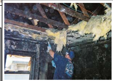
Rich Segally rips out the ceiling.
