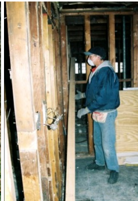
Wayne Kozak prepares studs to install drywall.
