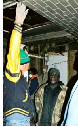
Tim Malloy discusses ceiling repair options with Ronnie, the homeowner.
