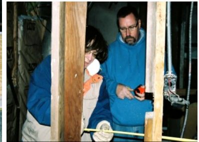
Mary Anne Koke and Keith Burke measure space to install cabinets.
