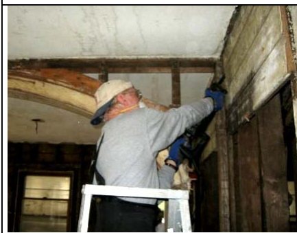
John Herr saws tongue and groove siding after removing plaster off Gerry's living room wall.
