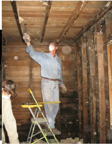
Warren Opperman completing the gutting of Gerry's kitchen.
